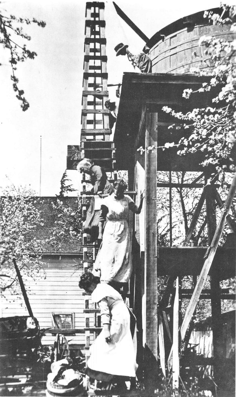
Water tanks served as personal reservoirs for valley families and were a common part of the landscape in the early 1900's. They also served as an excellent viewing platform as illustrated in this 1912 photo by J.O. Tucker.
