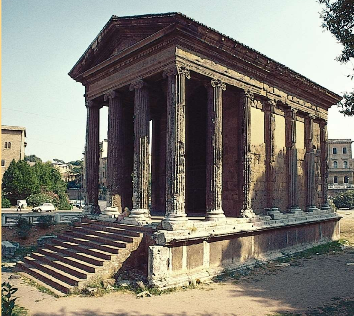
Temple of Portunus (god of harbors), Rome, Italy, ca. 75 BCE. Stone (originally overlaid with white stucco in imitation of Greek marble)
