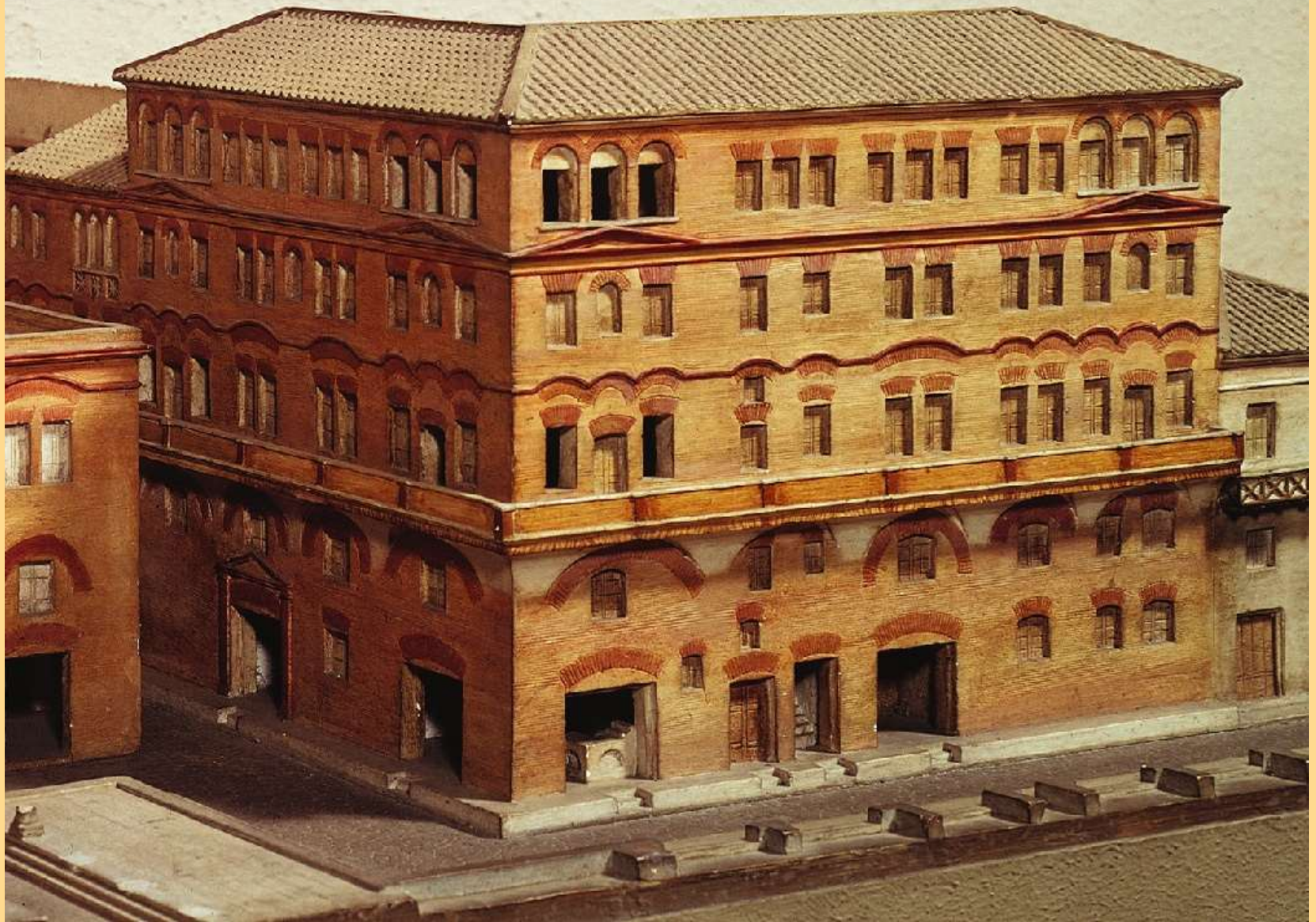
Model of an insula, (pl. insulae) Ostia, Italy, 2 nd c. CE. Originally: Brick faced concrete Museo della Civiltà Romana, Rome.
